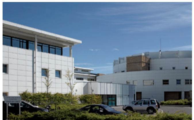
Figure 8 Health care building Scotland using light steel (Image courtesy of BW Industries Ltd)
