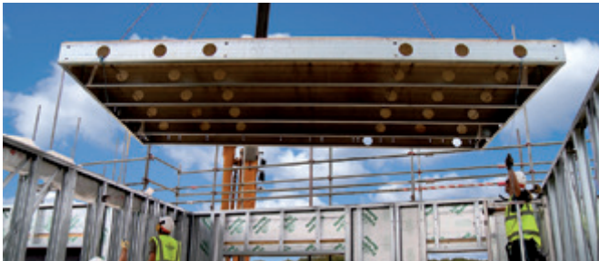
Figure 7 Light steel floor cassette (Image courtesy of Kingspan Profiles and Sections)
