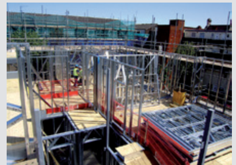
Light steel in residential building
