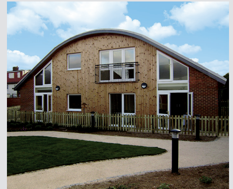
Code Level 5 modular houses in west London
