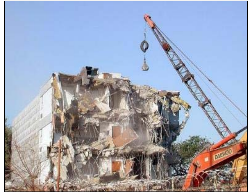
Demolition and crushing (downcycling)
