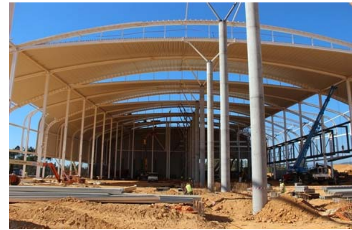
Deep decking system (Portugal)
