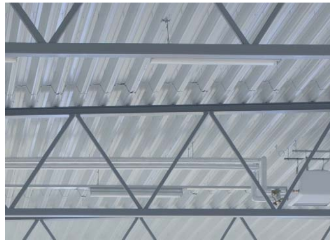
Long span roof claddings (Finland)
