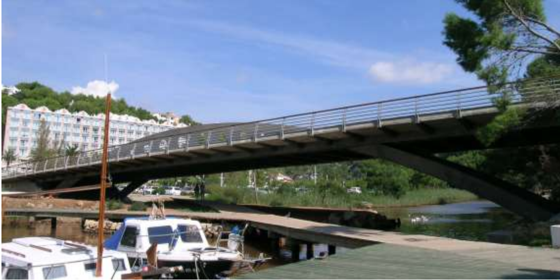
Figure 1. Minorca Duplex Stainless Steel Bridge.
