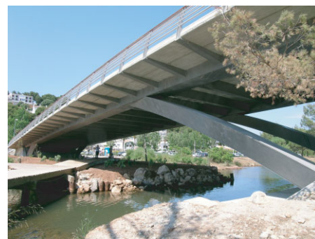
Fig. 4: View of bridge from below
