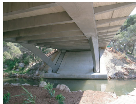
Fig. 2: Abutment 2. view of the completed element
